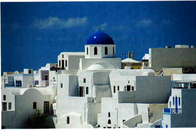
Fig. 3. The thick white walls and roofs of Santorini prevent unwanted heat from entering during the hot summers.
