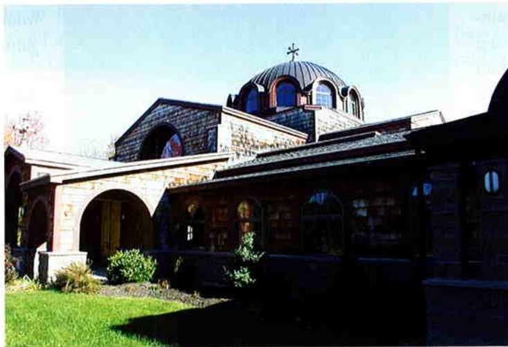
Fig. 1. Operable windows in the dome and elsewhere allow St. Demetrios in Saco, ME, to naturally “breathe,” saving energy and providing a more comfortable environment for parishioners.
